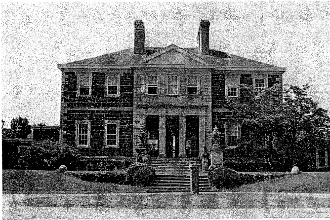
Fig. 12. Mount Airy, north facade. (Photograph by Dell Upton.)
